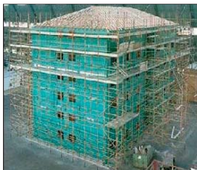
Fig 2. Six-storey TF2000 timber framed structure built by TRADA/BRE at Cardington 1995-2000
